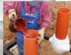
Sleeve pipe filling PLASTELEN®-KS Hot Casting Compound
