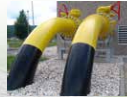
Ground to air transition LIQUITOL®-FK2 LIQUITOL®-FK2 C
