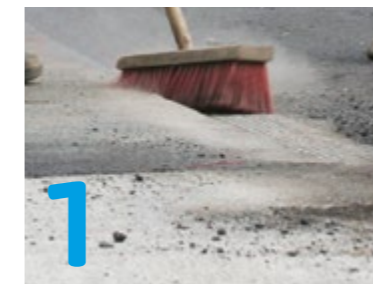
1 Clean the joint edge and dry if necessary
