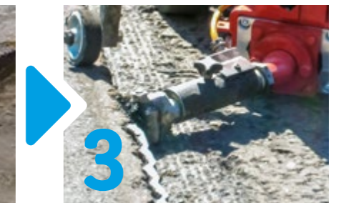
3 Use the TOKOMAT® to extrude the joint compound directly onto the edge
