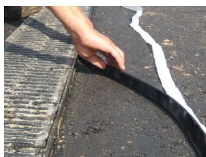
TOK®-Band SK used on drainage channels in asphalt surfaces.
