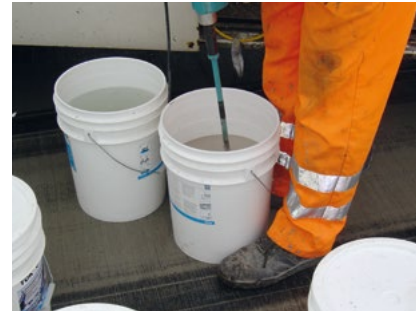
Mixing TOK ® -Crete 45 V2.0 is mixed with water (20 kg = 1.2 litres of water).
