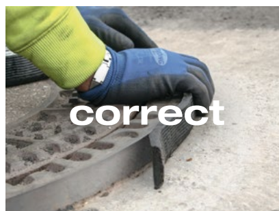
TOK®-Band SK used on hydrant and valve caps and the adjoining asphalt surface.
