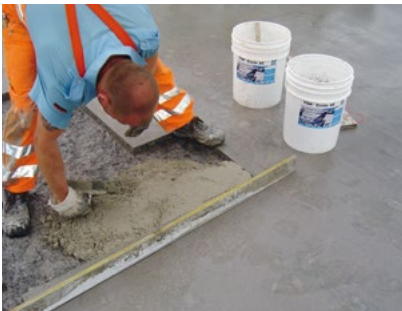
Installation Then install quickly as the pot life is 10 minutes.
