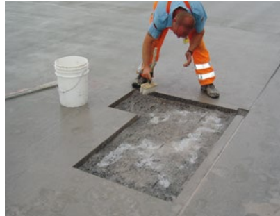
Preparation The prepared surfaces should be moistened. Priming is not required.
