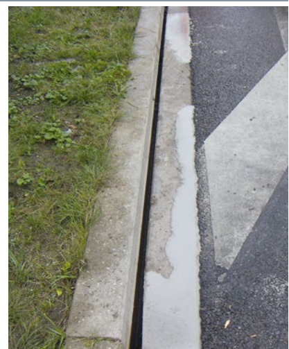
Repair is ready Pack up. Finished.
