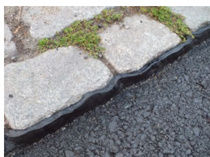
Joint formation at curb gutters using TOK®-Band SK or applied with the TOKOMAT®.
