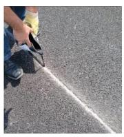
surface grip, it is necessary to sprinkle the compound with an excess of grit after it has been poured. For this, we recommend a grit with a PSV value (Polished Stone Value) of 40 to 60, grain size approx. 0/5. It is vital to ensure that the grit is dry when applied. If the grit is damp, the fresh
