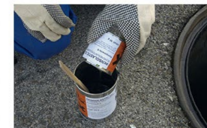
Mixing Stir component A well before processing, then add component B.
