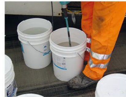
Mixing TOK®-Crete 45 V2.0 is mixed with water (20 kg = 1.2 litres of water).
