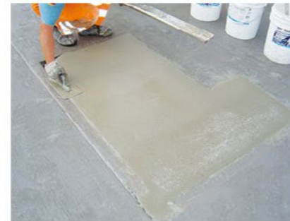
Smoothing The smoothing or removal of any excess must be done immediately. After 8 hours a compressive strength of approximately 30 N/mm 2 is reached.
