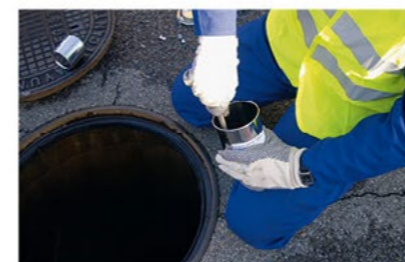
Stirring Mix the two components with the supplied rod (approx. 60 seconds). Pot life of the material at +23 °C (+73.4 °F): approx. 4 min. The pot life reduces with increased temperatures.
