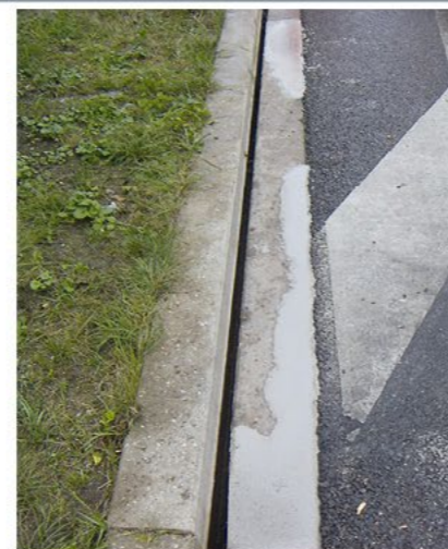
Repair is ready Pack up. Finished.
