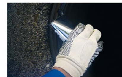
Pour out After mixing, the compound is evenly distributed on the support edge.
