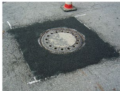
Sprinkling Then sprinkle the surface (e.g. blast furnace slag or coloured quartz sand) to ensure good surface grip. The colour of the sprinkling material determines the colour of the finished coating.
