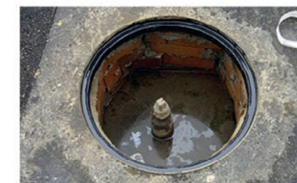
Allow to dry Depending on the weather and the temperature, wait approx. 10 to 20 m until the compound has dried but has not yet cured (finger test!).
