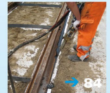
Track construction and civil engineering
