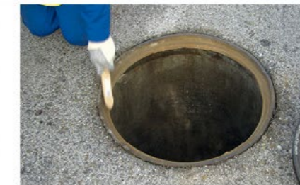
Remove any rust from the surface of the supporting edge with a steel brush and then wipe dry.
