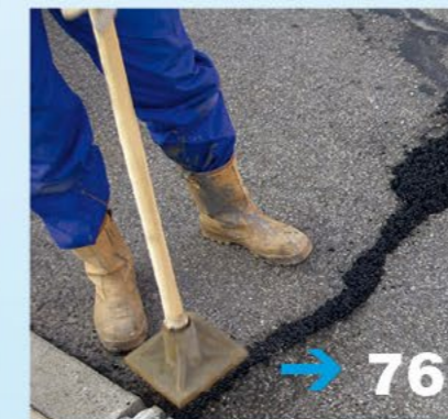
Repair asphalt
