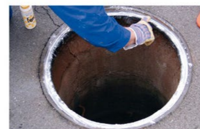
Sprinkle with talcum powder It is recommended to sprinkle the surface with talcum powder to help prevent the cover sticking to the manhole ring.
