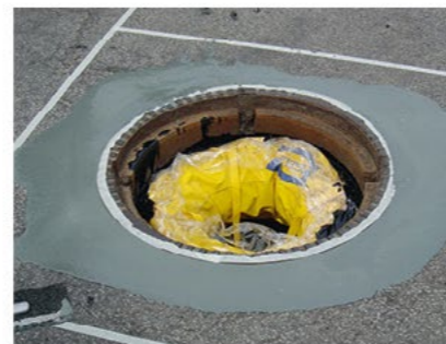
Apply Finally, apply the compound. It is possible to repeat the application.
