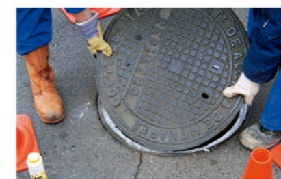
Put the cover back on. Then replace the manhole cover. Pay attention here to the correct timing between applying the compound and placing the cover to achieve the desired effect.
