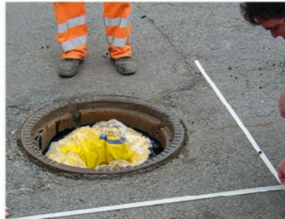
Masking surfaces Mask the surfaces to obtain a clean overall appearance.
