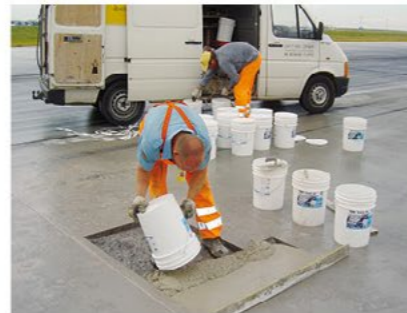
Installation It is recommended that 2 people work on larger projects so that "fresh on fresh" can always be installed.
