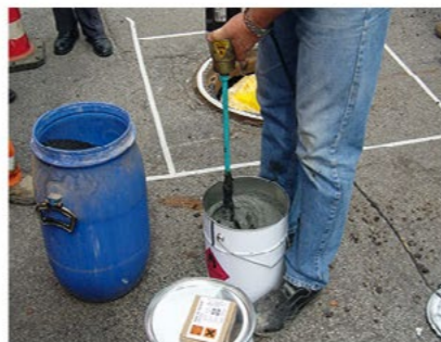
Mixing Stir up the coating compound. Then add the hardener and mix well. If required, fill with quartz sand somewhat to pre-fill large uneven surfaces.
