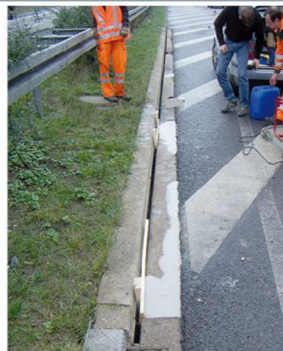
Shuttering and installation Shuttering, mix up the material, install. Wait a short period of time. Remove the shuttering.
