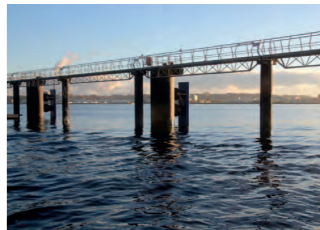
Germany, Port of Kiel, Ostseekai MarineProtect®-2000 FD Pier protection on the largest cruise ship dock, DN 2400 (96")
