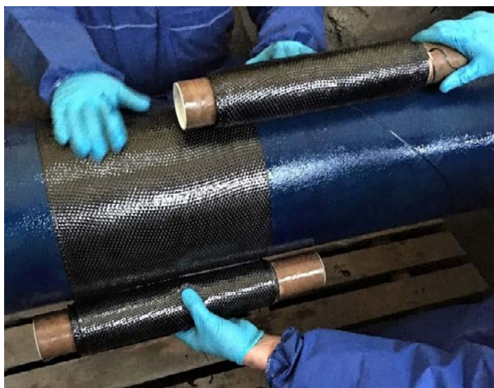
Figure 4. Easy application of DEXPAND-CF70.
